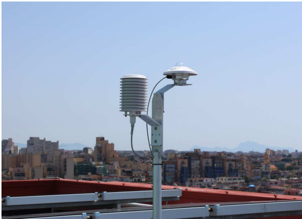
Fig. 10. Installed Pyranometer LP PYRA 02
