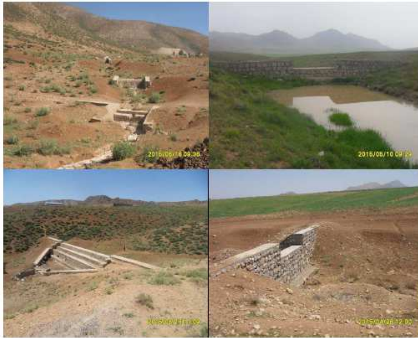
Fig. 3: The sedimentary rock dams for control of flood and sediment in Sardasht basin
