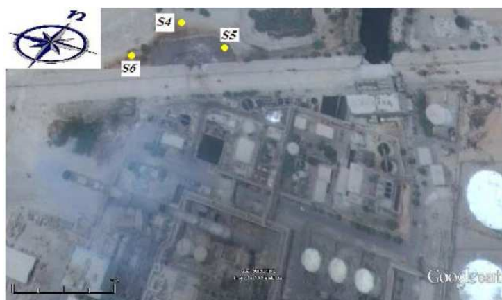
Fig. 3. The location of the pond in the north of ATPP and the location of soil samples around the pond
