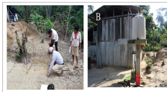
Fig. 1: Rainwater harvesting systems; (a) site selection; (b) water harvesting system installed; Source: Prolluvia Project (contract no. 185-2018-FONDECYT-MB-IADT-SE)
